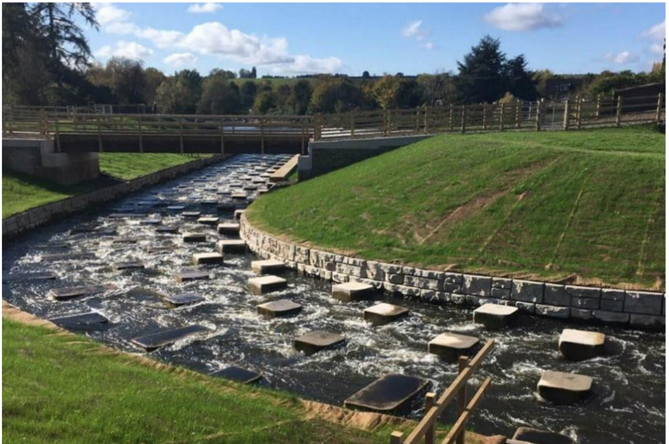
Figure 5: Perturbation fish pass on the River Severn
