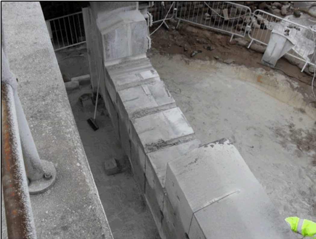
Figure D1 Weir being removed in 2015
