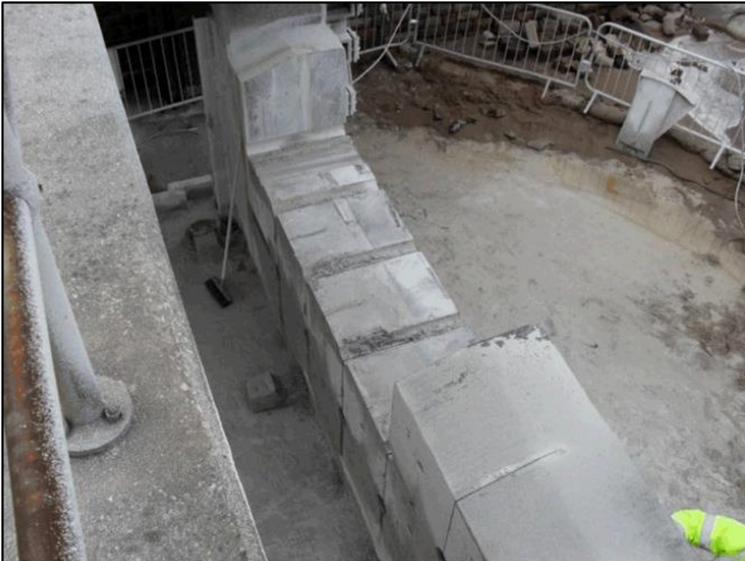
Figure D1 Weir being removed in 2015
