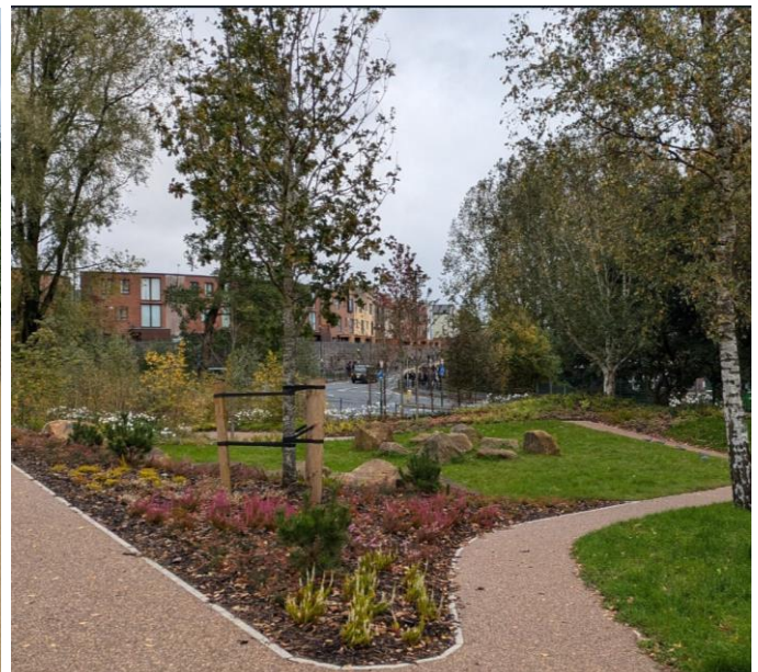
Rock Street, Oldham – SuDS enabled park with disability access, swales and raingardens
