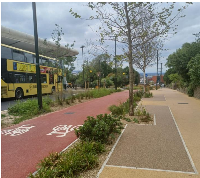
West Street, Oldham – Bioretention features with integrated cycleway
