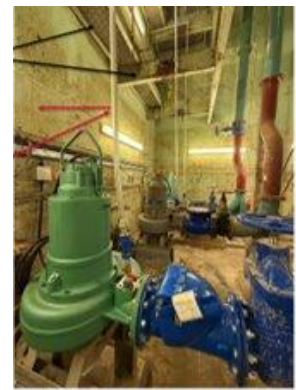
Image 1 & 2: Existing Pumps to be upsized.
