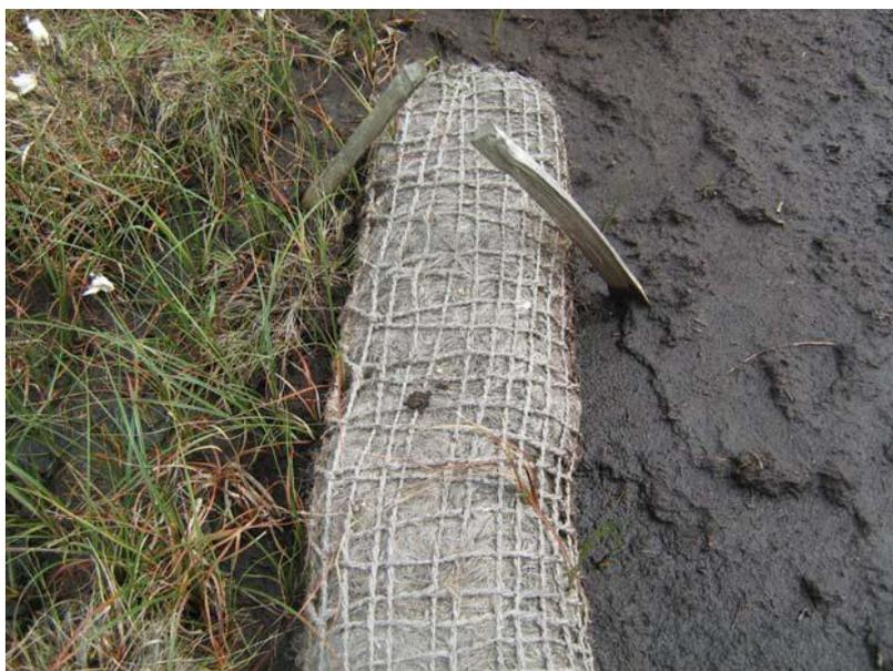
The innovative use of coir rolls to reduce peat wash-off and surface water runoff on the flatter bare peat pans is indicating that the installation of the coir rolls has allowed the peat surface to retain slightly wetter conditions on the bare peat pans and some evidence of peat wash-off being held back.
