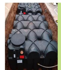
An attenuation tank and supply plumbed into the home can replace potable water for flushing toilets, laundry and irrigation.
