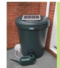
Smart water butts maximise rainwater reuse and minimise surface water and sewer flooding - automatically releasing water when it's likely to rain to create storage capacity for rainwater.
