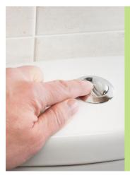
Dual flush or ultra low flush toilets are available with flushes as low as 1.5 litres per flush, compared to the UK average of 9 litres.
