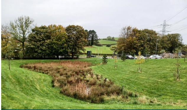
Basins - Infiltration and attenuation
