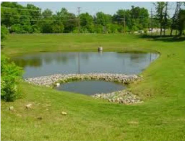
PHOTO OF STONE EMBANKMENT SEDIMENT FOREBAY
