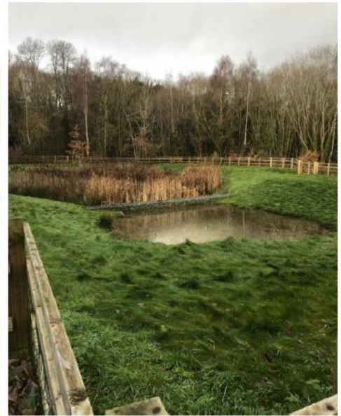
PHOTO OF CONCRETE SEDIMENT FOREBAY
