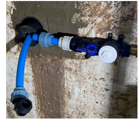
Example of a service pipe being ducted and insulated through a basement wall
