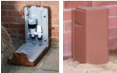
Wall mount box in situ and insu-duct
