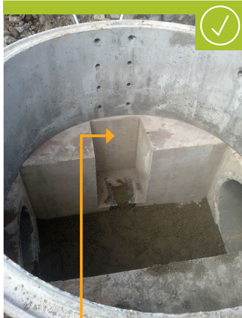
'Boxed out' benching positioned flush with manhole ring above.
