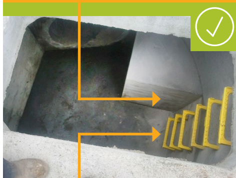
Step rungs in plumb and vertical alignment equally distanced apart.
