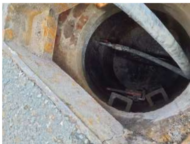
Figure 3: Grout injection to seal a manhole
